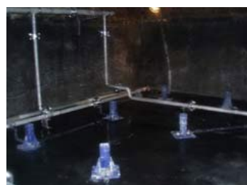
First class hotel Kitchen wastewater treatment pit Water purification and deodorization February 1999
