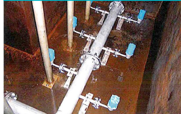
Piping support example
