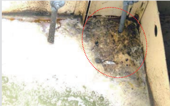
Diffusion irregularities occurred, and oil content accumulated in the corner, where maggots grew.
